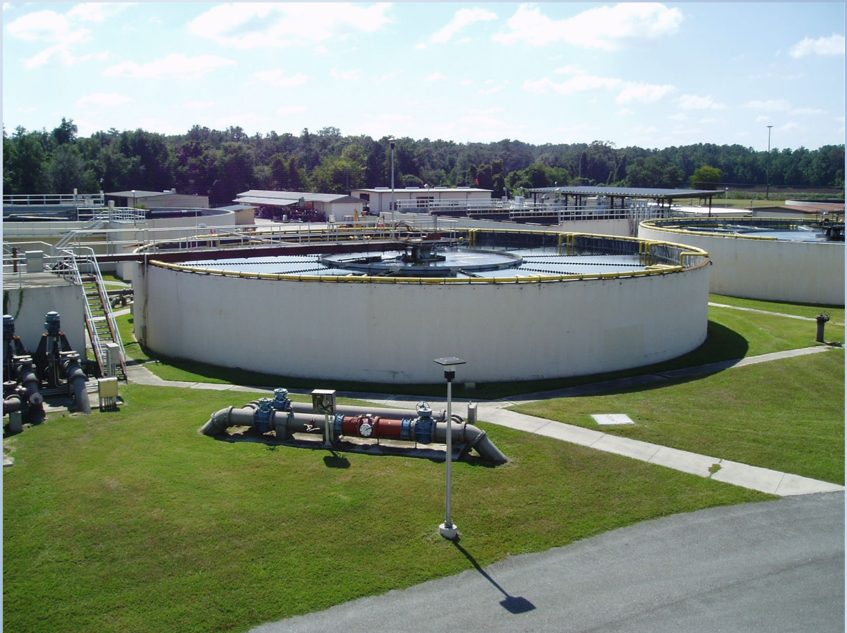
The clarifiers at the GRU Kanapaha facility
