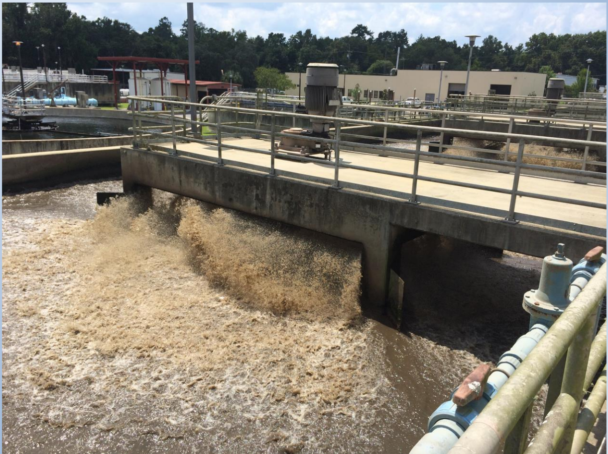
The aeration basin at the GRU Main St. Facility
