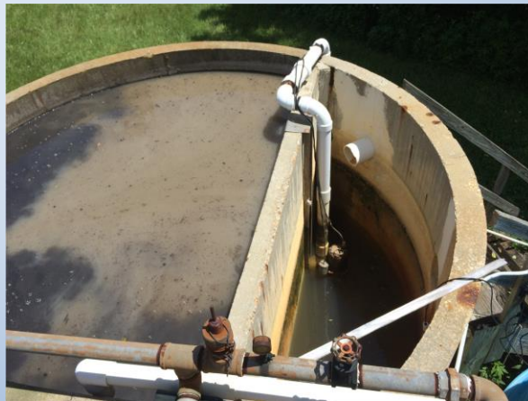
Camp Kulaqua clarifier and chlorine contact chamber
