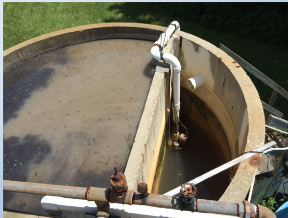
Camp Kulaqua clarifier and chlorine contact chamber
