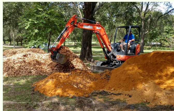
This photo shows the different materials that were put under the drainfield of the INRB system at Poe Springs County Park.
