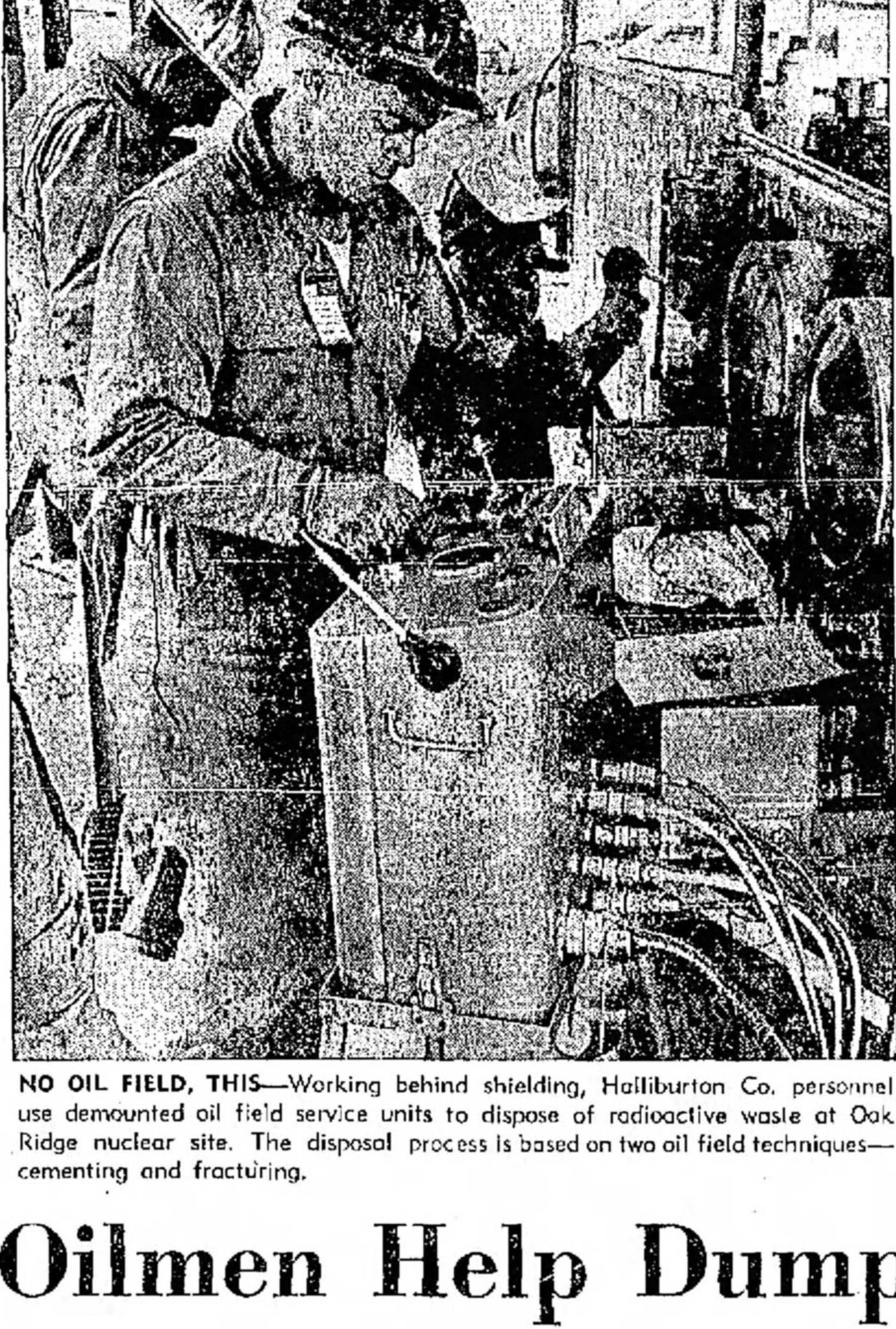
NO OIL FIELD, THIS—Working behind shielding, Halliburton Co. personnel use demounted oil field service units to dispose of radioactive waste at Oak Ridge nuclear site. The disposal process is based on two oil field techniques—cementing and fracturing.
