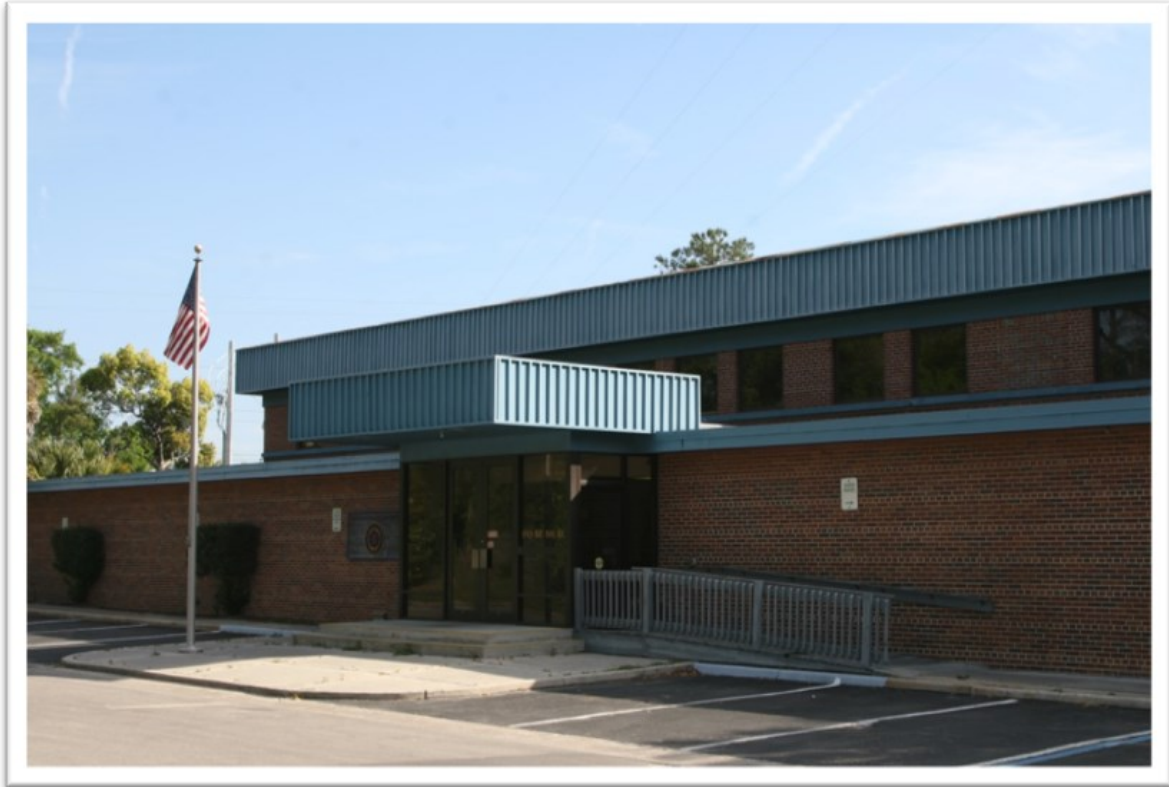
Fire Rescue Headquarters Building
