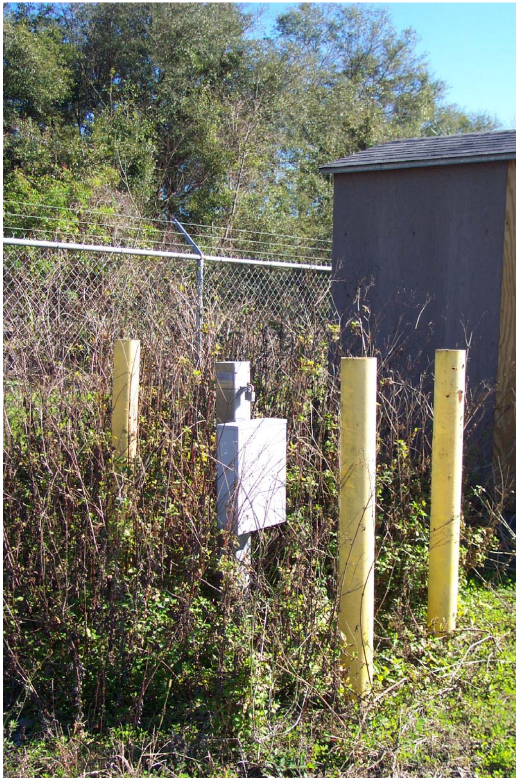
PHOTOGRAPH 5. CLOSE-UP TYPICAL MONITORING WELL, KOPPERS, 1 FEB 06
