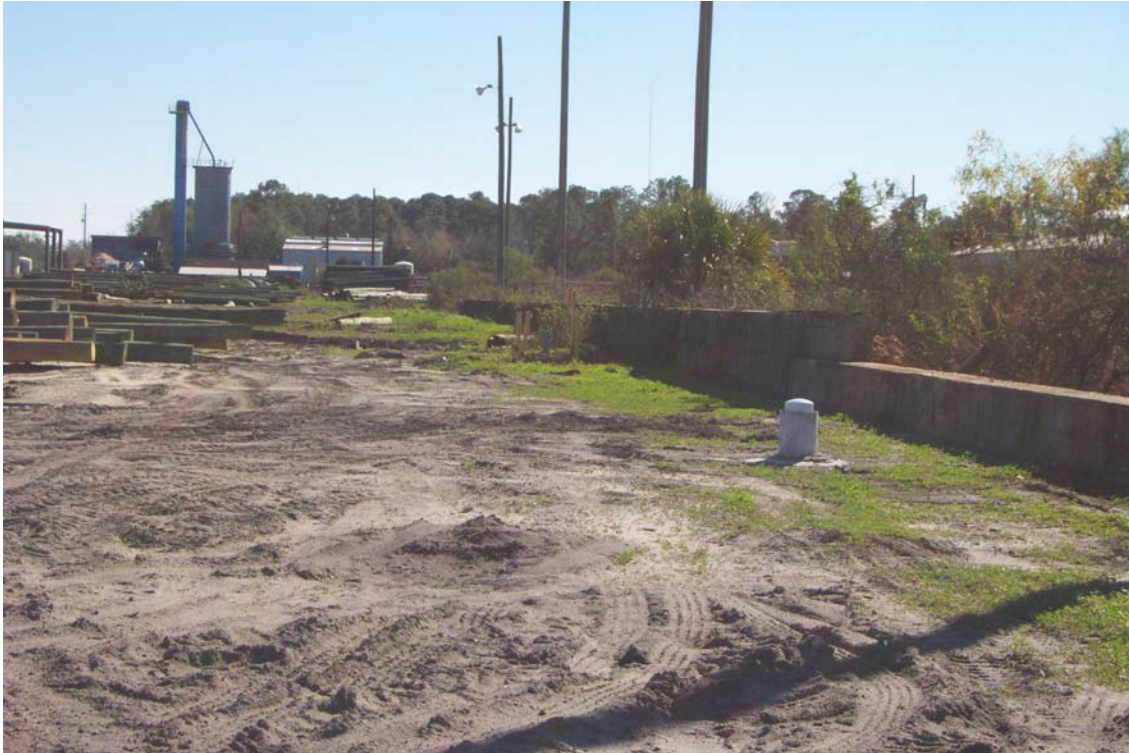
PHOTOGRAPH 10. CLOSE-UP, DRIP TRACK AREA, WITH NEW FLORIDAN WELL, KOPPERS, 1 FEB 06
