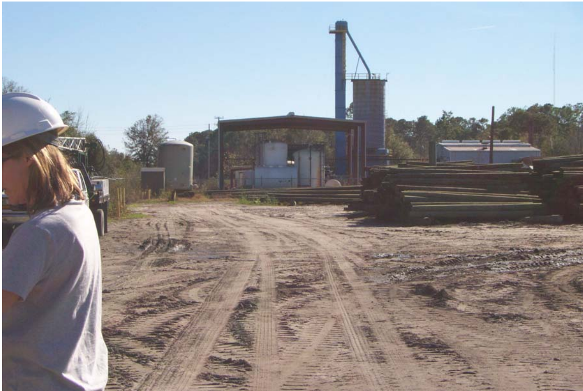
PHOTOGRAPH 6. WATER TREATMENT PLANT, KOPPERS, 1 FEB 06
