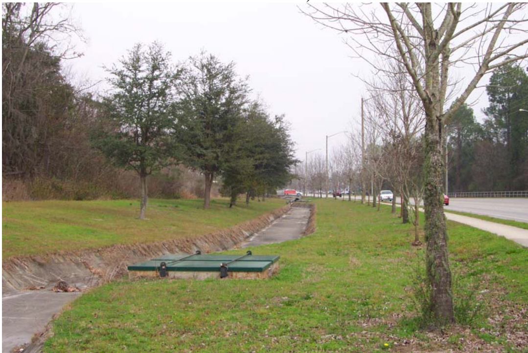
PHOTOGRAPH 17. SUMP, CABOT TRENCH, 2 FEB 06
