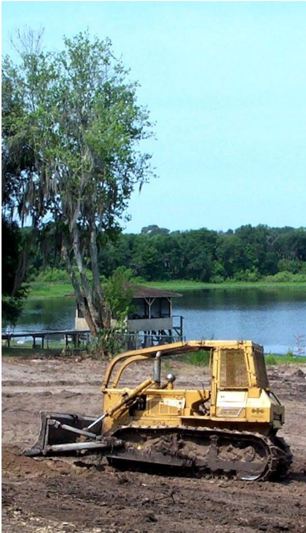
A dozer illegally clears vegetation on a lake. This is an example of a prohibited development activity.
