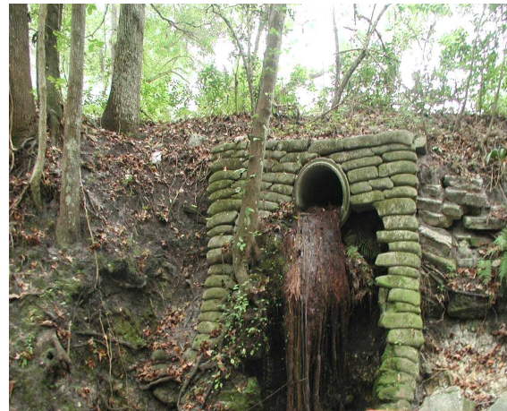
Eroded banks near a stormwater inflow
