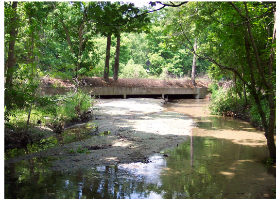
Sand filled culvert on Hogtown Creek at NW 8 th Ave
