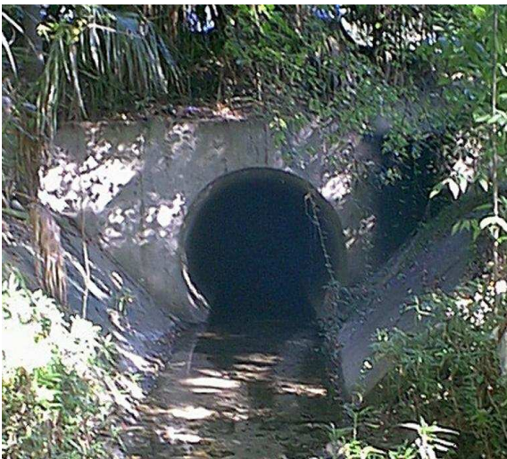
Tumblin Creek at the 60-inch culvert at Shands at AGH just north of SW 5 th Avenue
