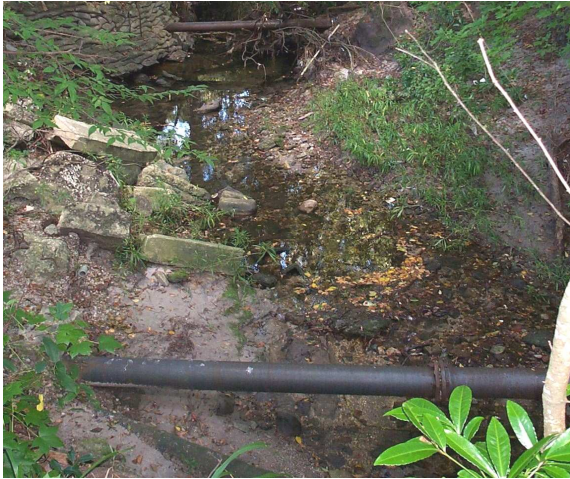
Sanitary sewer and gas lines that were originally laid below the streambed of Tumblin Creek
