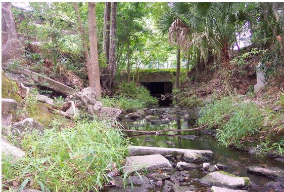
Concrete rubble in Tumblin Creek at P. K. Yonge School
