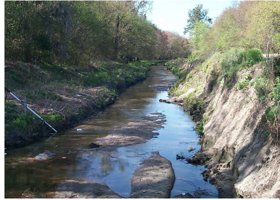
Sand deposition in the dredged channel of Tumblin Creek west of US 441
