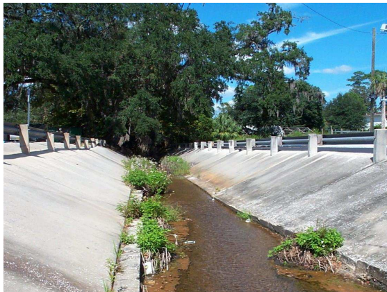
Tumblin Creek flowing through a concrete channel behind Subway at US 441
