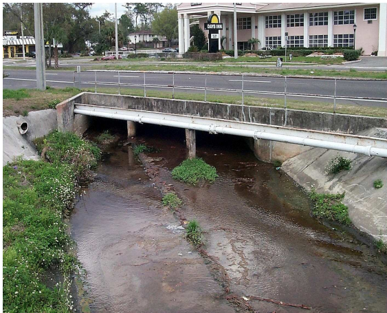
Stormflow on Tumblin Creek at US 441
