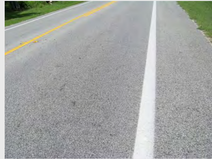
County Road 241, Resurfaced 2002
