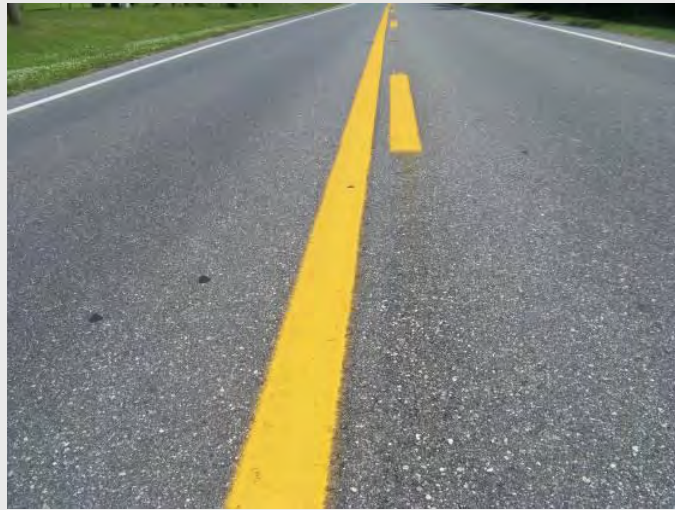
County Road 241, Resurfaced 2002
