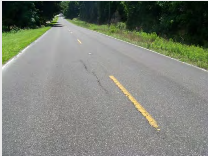
NW 94 th Avenue, Paved 1979
