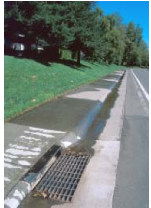
Discharge of nutrient-laden irrigation water to the stormwater system
