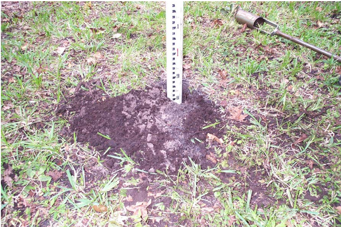
Image 26. Soil Boring 7, Depth of Soil Boring
