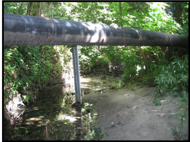
Wastewater Line Crossing Tumblin Creek at TUMSW5
