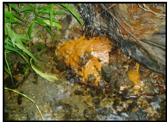
Orange Growth, Likely Iron Bacteria, at Spillway Outfall with Elevated Fecal Coliform Concentrations (TUMBPDs)
