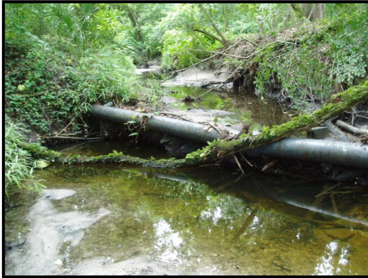
Wastewater Line Crossing Rattlesnake Branch
