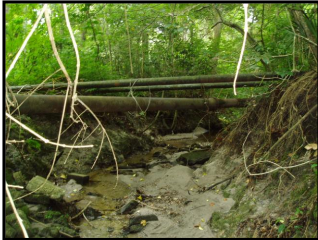
Water and Wastewater Lines Crossing Over Elizabeth Creek
