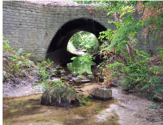
North branch of Little Hatchet upstream of culvert
