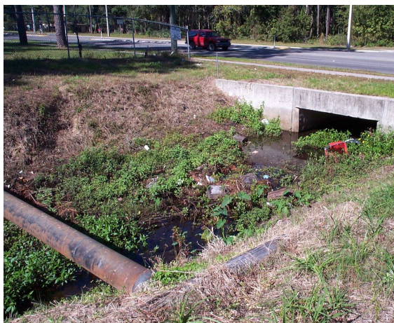
Sanitary sewer line above Lake Forest Creek at SR26.
