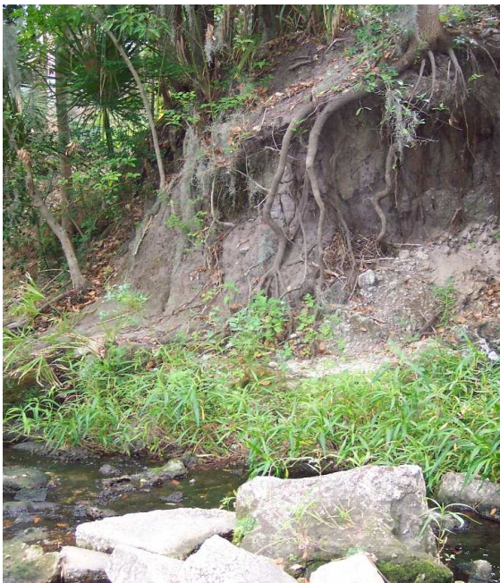
Erosion and bank failure on Tumblin Creek at P.K. Yonge School.
