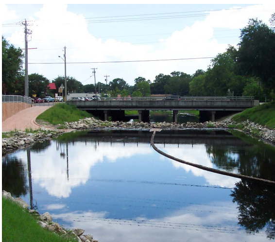
Hogtown Creek sediment trap upstream of NW 34th Street (facing west).
