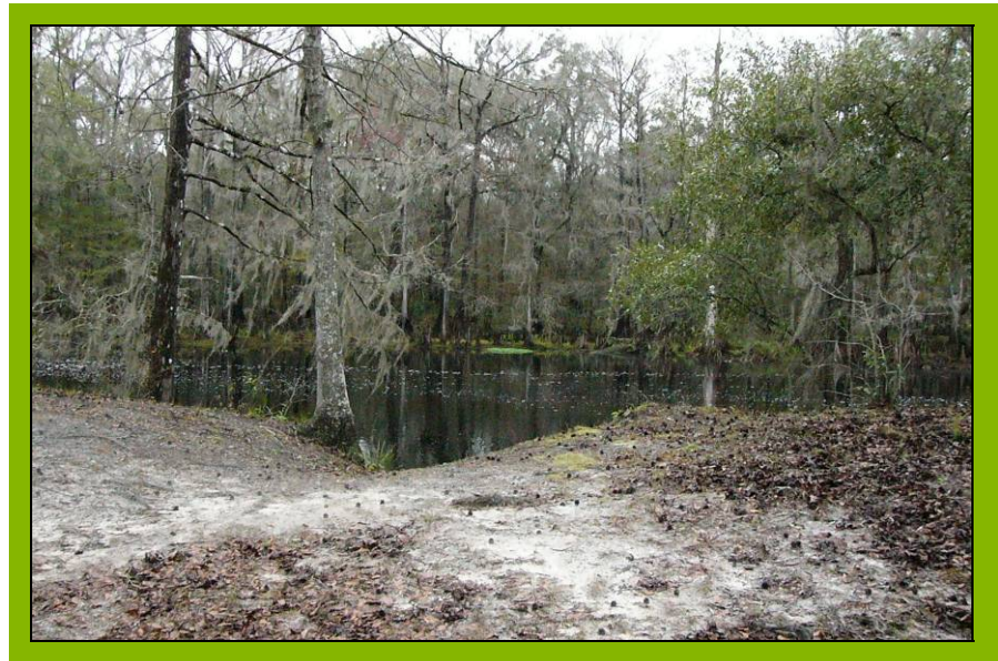
Barren river bank area & erosion; note contrast with heavy natural vegetation on opposite bank
