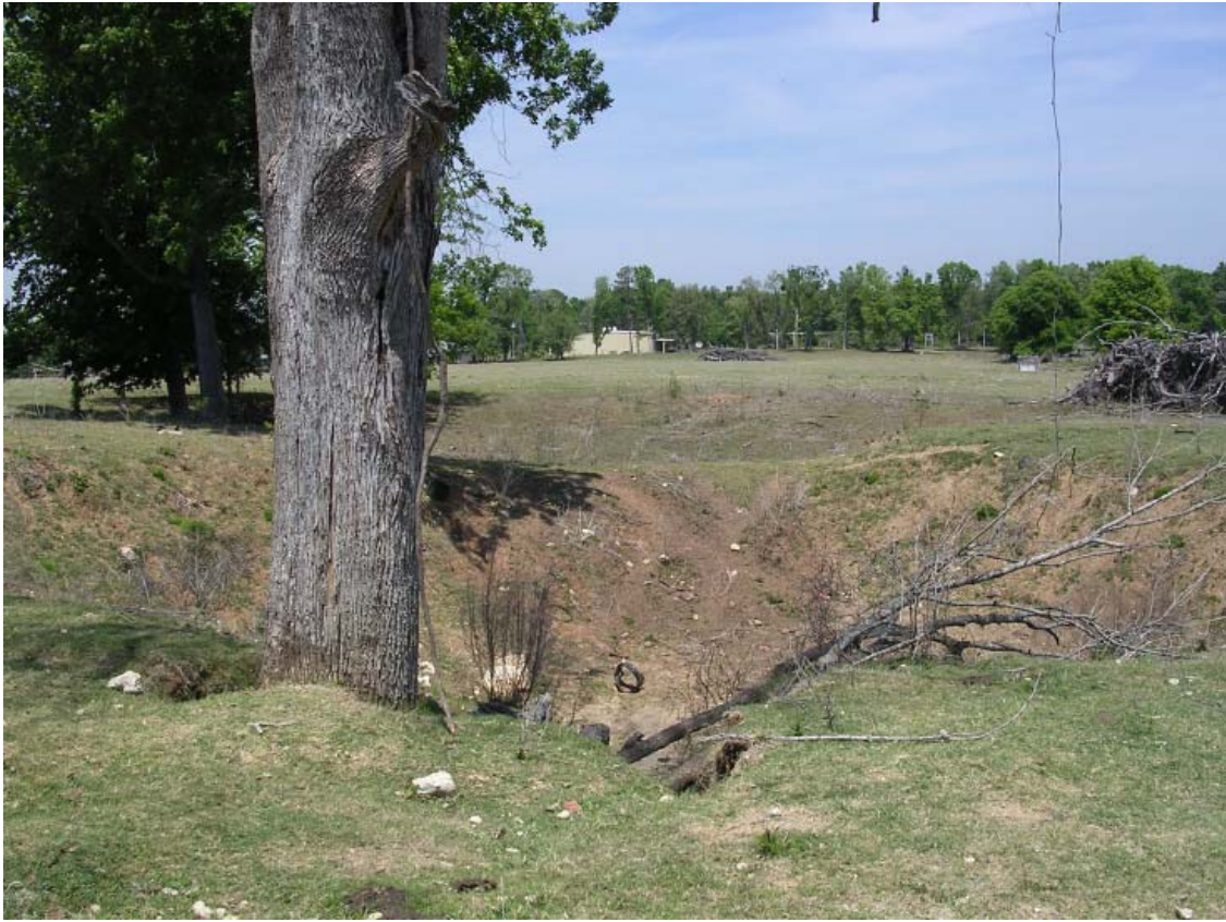
Plate 7. Sinkhole above and in the vicinity of the Terminal Room of the Mill Creek Sink Cave.
