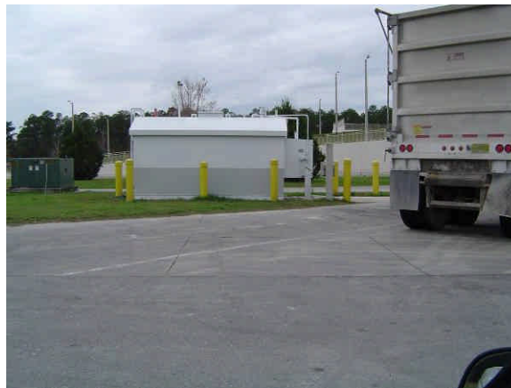
Fleet fuel facility at the Transfer Station in the Leveda Brown Environmental Park
